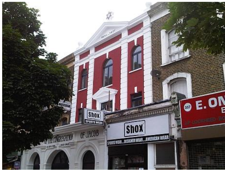
The newly restored classical frontage of the Congregation of Jacob Synagogue, made possible through funding from members of the synagogue and the Veolia Charitable Trust (2010)
